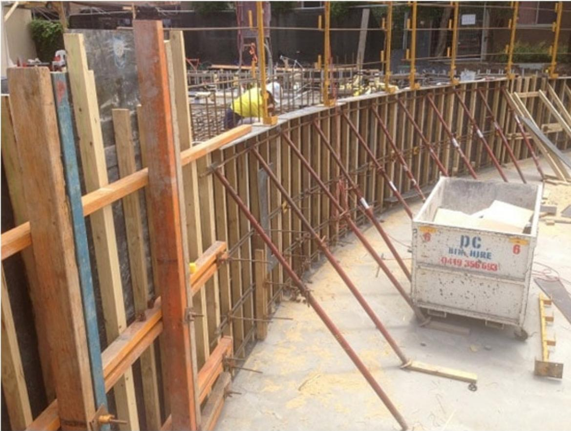
Conventional Formwork (Source: Fine Line Construction Services)
